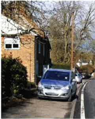
Pavement obstructed along Cambridge Road, Quendon.
