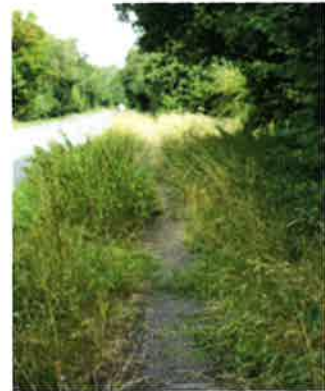
Pavement along B1383
